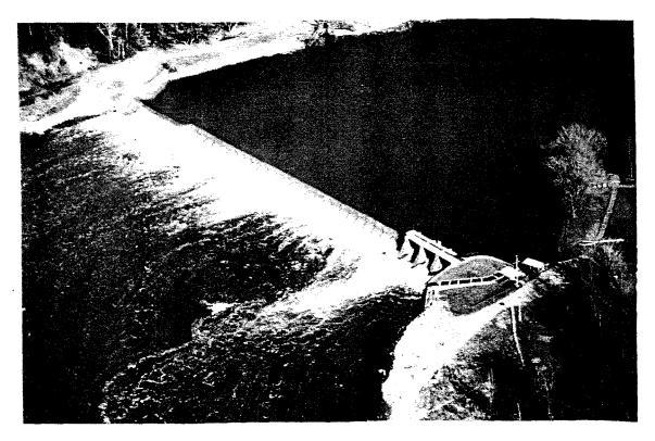
8. Sea lamprey barrier dam on the Saugeen River, Lake Huron, Ontario. This is the first barrier dam constructed in Ontario. It is a large multi-purpose dam, 180 m long (600 ft) and 2.7 m high (9 ft), built in 1969-70 with federal-provincial funds. A fishway and a lamprey trap are included.
