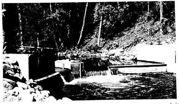
13. Sea lamprey barrier dam on Kaskawong River, Lake Huron, Ontario. A low head barrier dam constructed in 1980-81 of concrete. It has a built-in lamprey trap and jumping pool.
