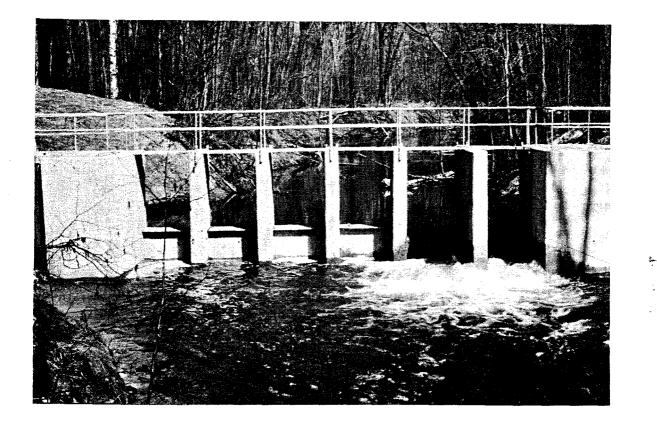
21. Sea lamprey barrier dam on the East **Branch** of AuGres River, **Lake** Huron, Michigan. A low head concrete dam constructed in 1983 with 2 stop-log bays to permit **drawdown**. In 1986 a coffer dam was constructed **downstream** to elevate the tailwater level and a jumping pool was added in the area of the stop log bays to facilitate fish passage. It has facilities for attaching portable **assessment** traps.
