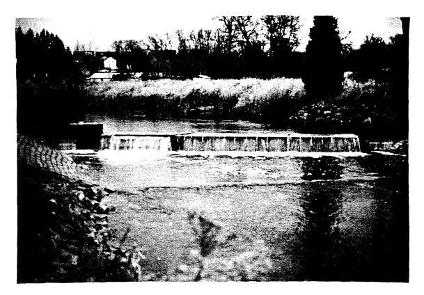
4. Sea **lamprey** barrier dam on Graham **Creek, Lake** Ontario, Ontario. It is a **low** head barrier dam **constructed** of steel sheet piling in 1983 **and** has a built-in lamprey trap and **jumping** pool.
