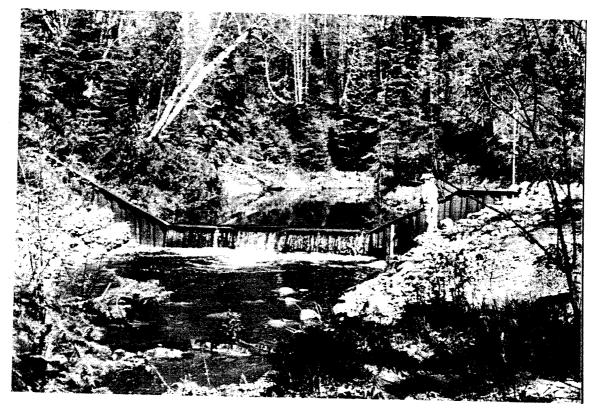
19. Sea lamprey barrier dam on Gimlet Creek, Lake Superior, Ontario. It is **one of** the earlier low head barrier dams constructed in 1979-80 of steel sheet **piling and** has a jumping pool, but mtatrap for lamprey.
