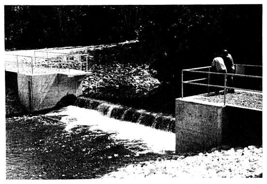
27. Sea lamprey barrier dam on the Misery River, Lake Superior, Michigan. A low head barrier dam constructed of concrete in 1984 with a slidegate to permit drawdown. It has a jumping pool and portable assessmenttra~. Note: Photograph for site No. 28 (East Twin River) is not included.
