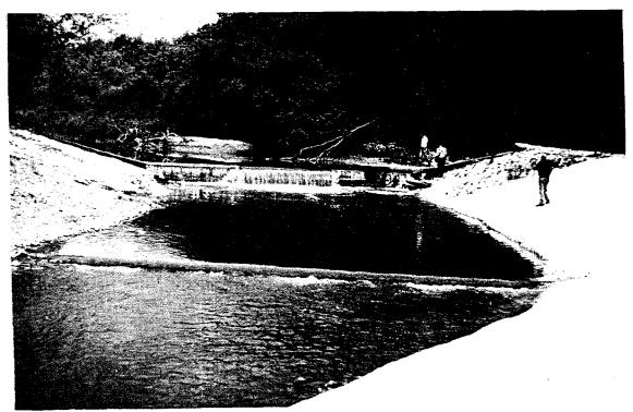
5. Sea lamprey barrier dam on Duffin Creek, Lake Ontario, Ontario. It is a low head barrier dam constructed of steel sheet piling and has a built-in lamprey trap and jumping pool. Note the structure downstream from the barrier to elevate and maintain the head of the jumpiqpool.
