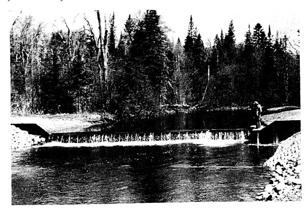
18. Sea lamprey barrier dam on Carp River (Sable), Lake Superior, Ontario. A low head barrier dam **constructed** with steel sheet piling in 1983. It has a built-in lamprey trap and jumping pool.
