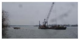
Figure 12 Construction of Rock Berms at E. River Marsh
